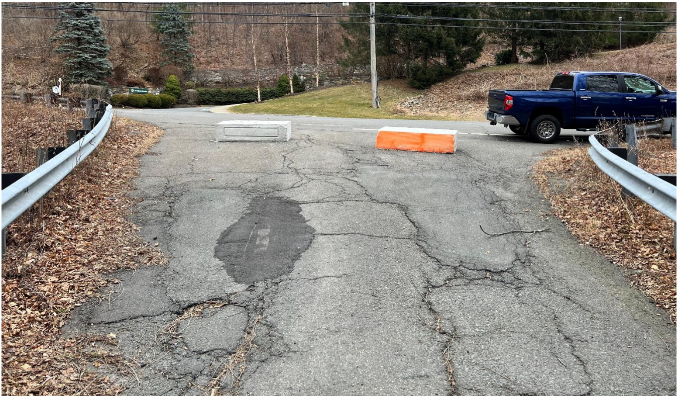
Photo Number: 2 East approach from bridge. Photo Taken: 03/14/2025
