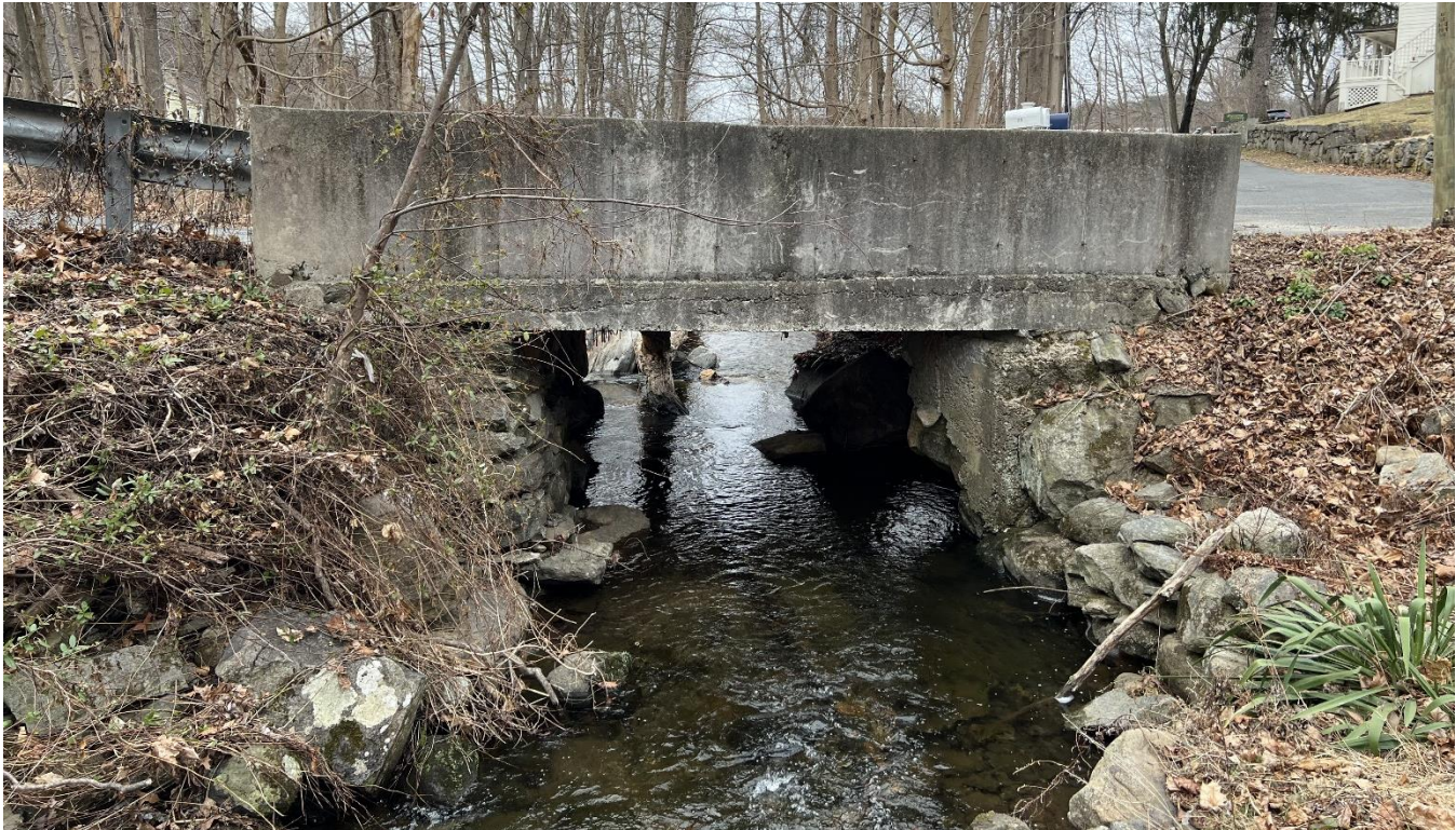
Photo Number: 5 North (upstream) elevation. Photo Taken: 03/14/2025
