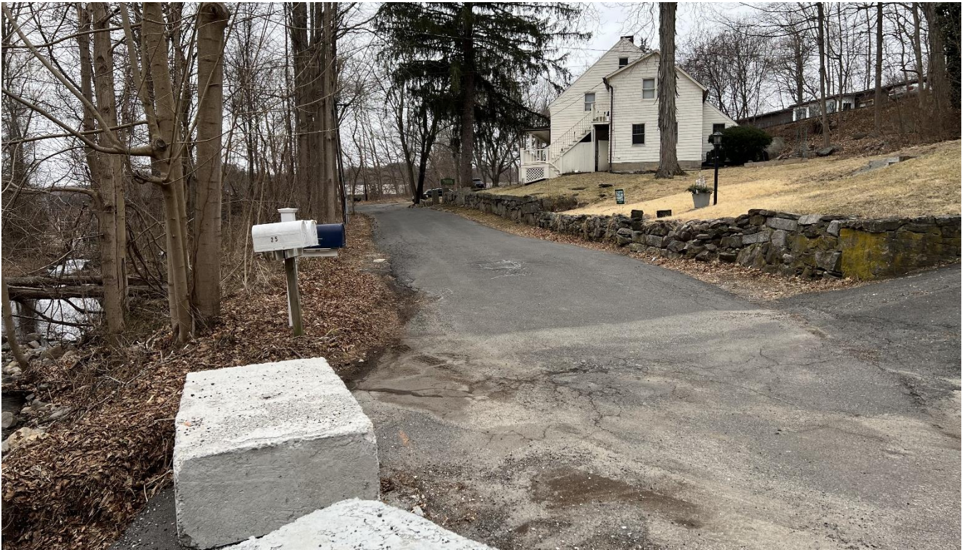
Photo Number: 4 West approach from bridge. Photo Taken: 03/14/2025
