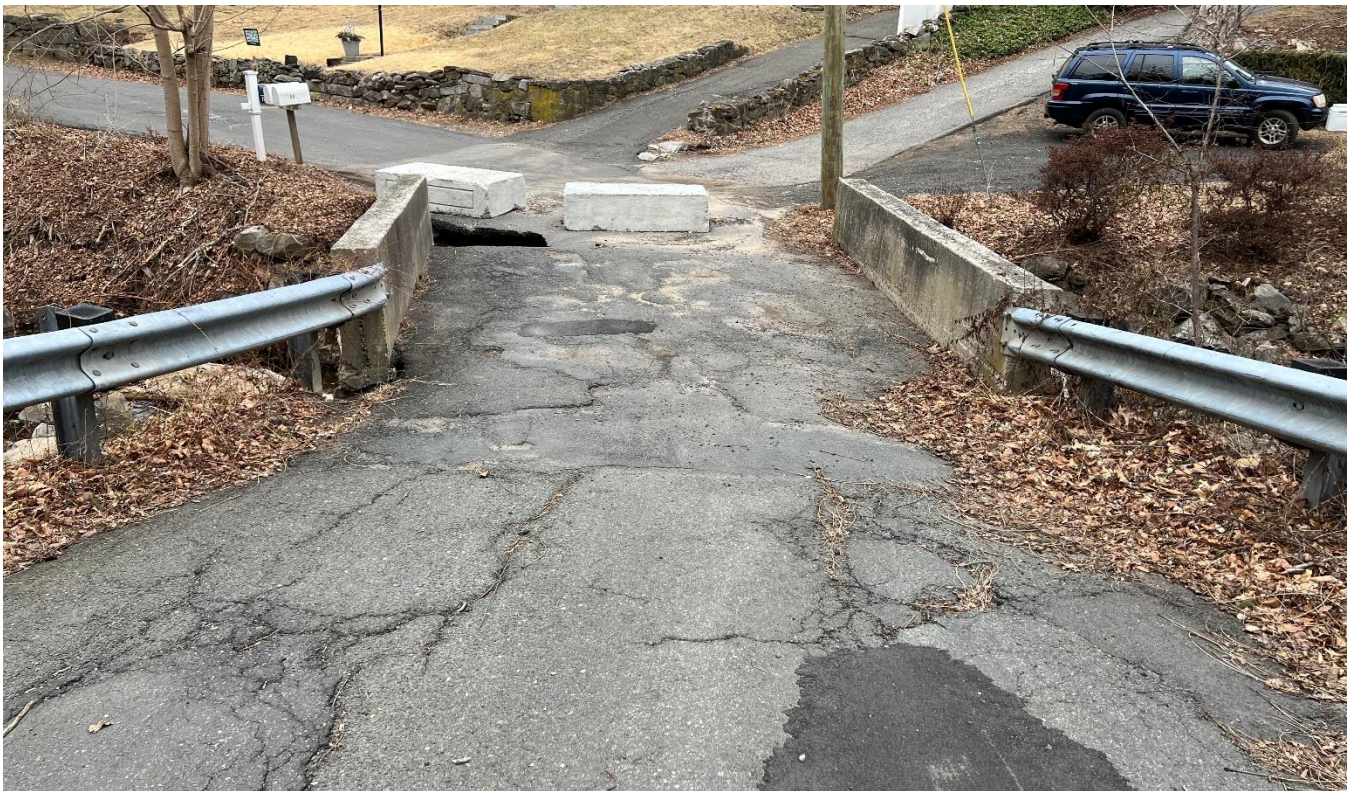
Photo Number: 1 Bridge from east approach. Photo Taken: 03/14/2025
